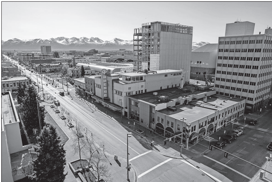
The 4th Avenue Theater in downtown Anchorage is photographed in May.
